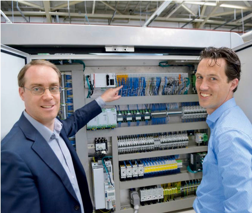
MetalFAB1 control cabinet with automation components from Beckhoff. (left to right) Jurjen Verhoeff, Account Manager at Beckhoff Netherlands and Mark Vaes, CTO at Additive Industries
